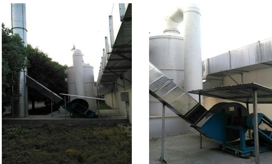
Figure 3 Rectified odour collection facility in Hefei in Anhui Province
