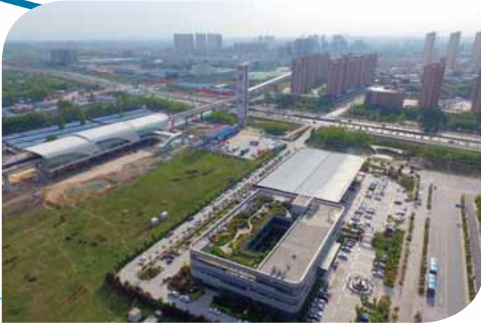
The extension of subway line 2 passing through CSC Zhengzhou has commenced trial operation 貫通鄭州華南城的地鐵2號線延長線已開始試運營
