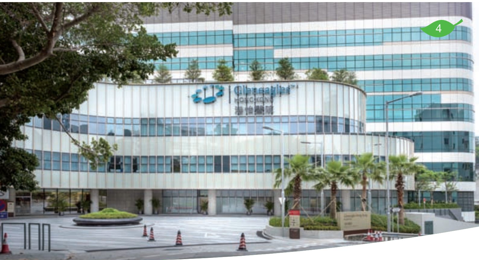
3 German Swiss International School Redevelopment, Phase 5 德瑞國際學校第五期重建工程
