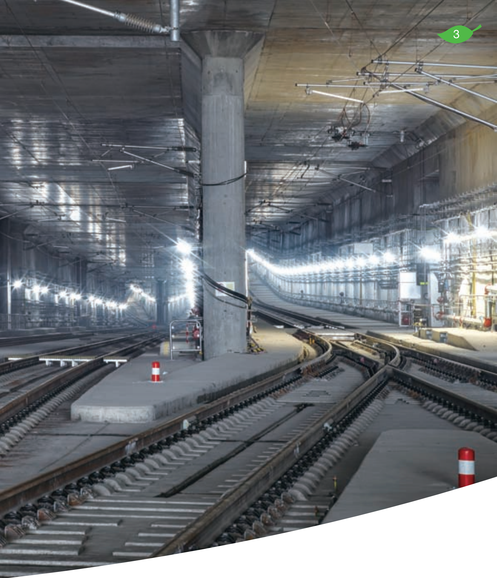
3 MTR Contract No. 830 – Guangzhou-Shenzhen-Hong Kong Express Rail Link (Hong Kong Section): Trackwork and Overhead Line System 港鐵合約編號830－廣深港高速鐵路(香港段)：軌道及接觸網系統
