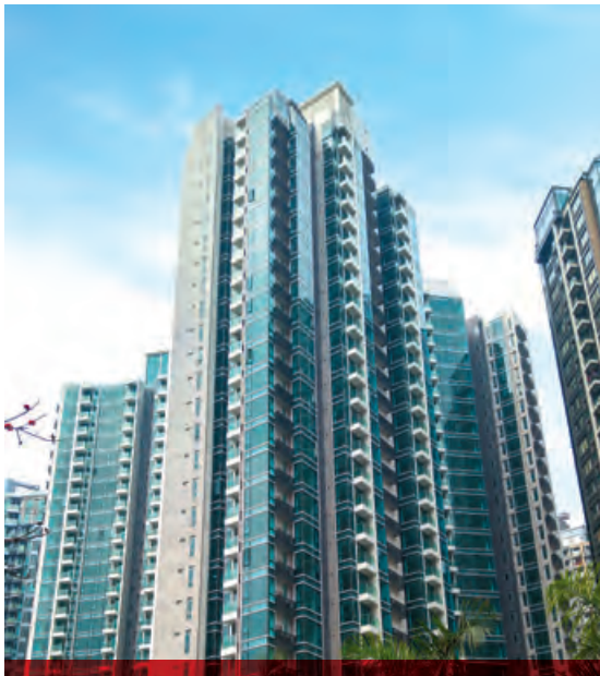
Aluminium window, sliding door, aluminium cladding and curtain wall for residential development at No. 18 Tong Chun Street, Tseung Kwan O 將軍澳唐俊街18號之住宅發展項目之鋁窗、趟門、鋁飾板及幕牆
