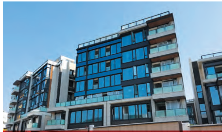
Aluminium window, door and aluminium works to towers for residential development, Kau To Shan, Shatin 沙田九肚山之住宅發展項目之鋁窗、門及大廈鋁製工程
