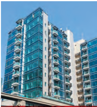
Tower curtain wall and podium façade for residential and commercial development at 33 Tong Yin Street, Tseung Kwan O 將軍澳唐賢街33號之住宅及商業發展項目之大廈幕牆及基座外牆
