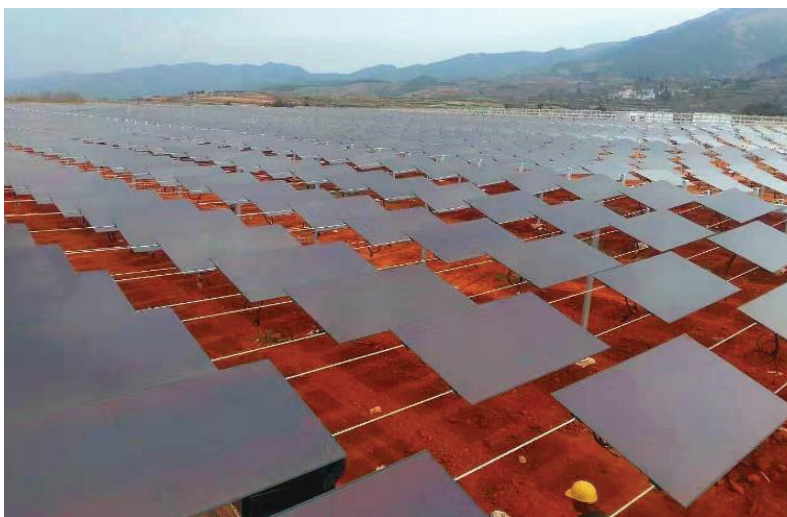
Photovoltaic Agricultural Poverty Alleviation Project in Xundian, Yunnan
