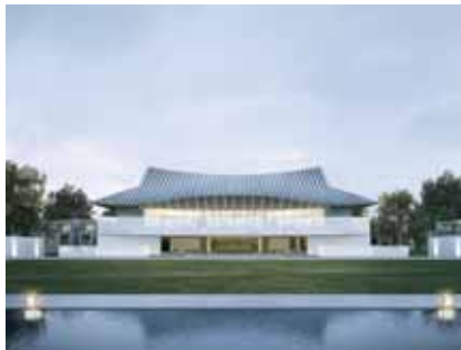
蘇州吳中區西山項目 Suzhou Wuzhong District West Mountain Project
