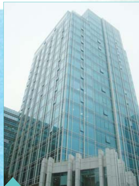
The Metropolis Tower was recognised in the Facility Management industry in Asia Pacific 都會大廈在亞太地區設施管理業內獲得認可
