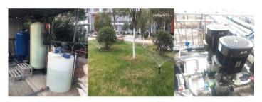
In order to make the most of water resources and reduce water wastage, the Company has set up a greywater recycling system, redirecting greywater to toilet flushing, landscaping ponds and landscaping sprinklers.
