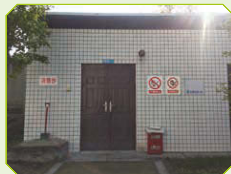
Fire Fighting facilities 消防設施
