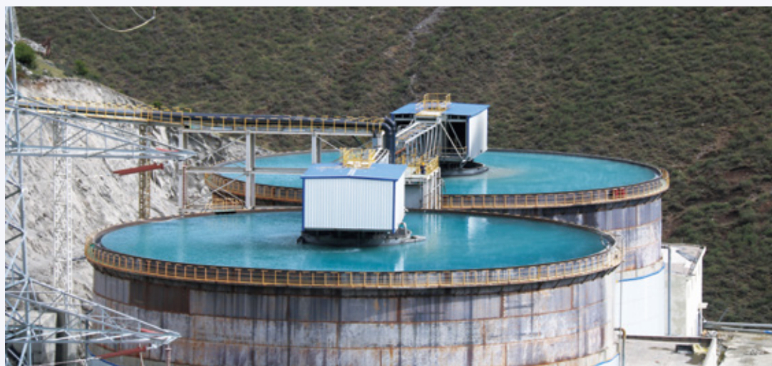
Jiama Mine's newly-built equipment
