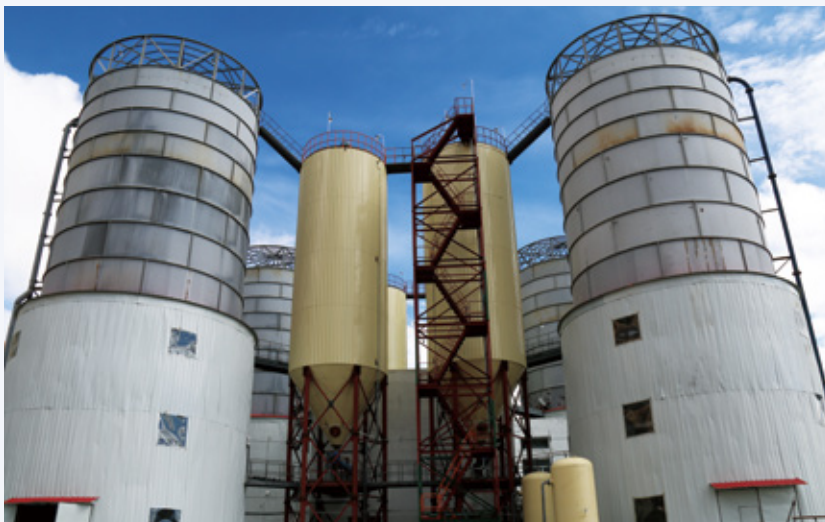
Backfill station at Jiama Mine
