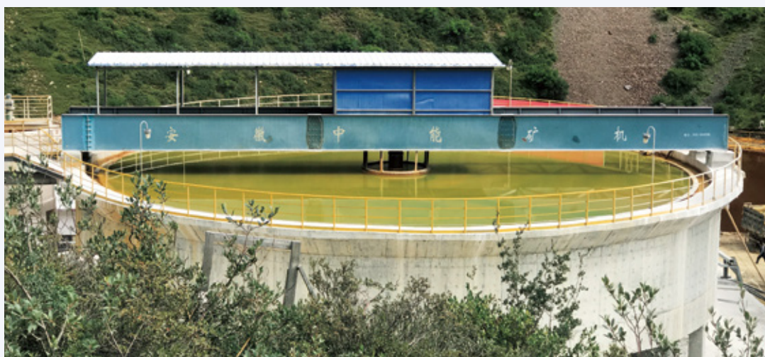
Jiama Mine invested 72 million yuan in constructing the sedimentation tank for iron removal of Sibuh acid spring water treatment plant
