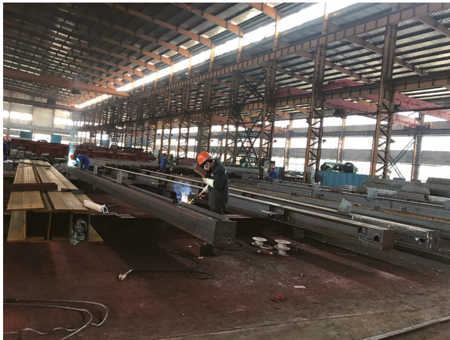
Staff are performing welding work 員工進行焊接工作
