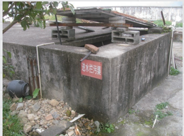
Wastewater filter and disposal system
