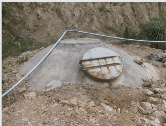
Self digestion enclosed pit for dead hog disposal
