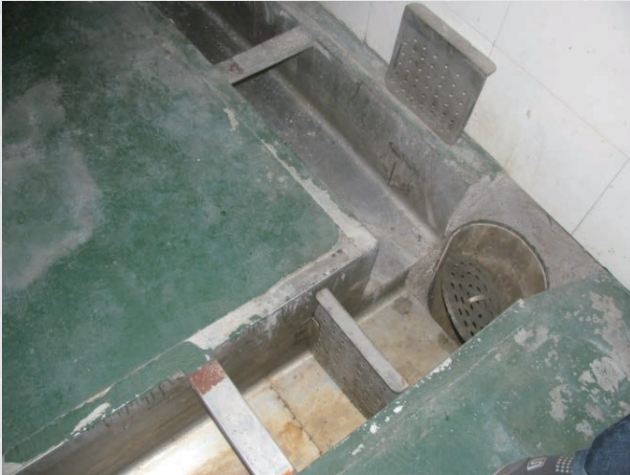
Gutters within slaughterhouse for waste water drainage
