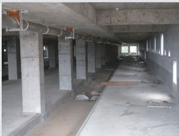
Construction of nullah within pig barns
