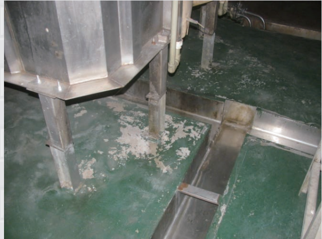
Gutters within slaughterhouse for waste water drainage
