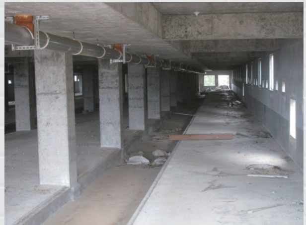
Construction of nullah within pig barns
