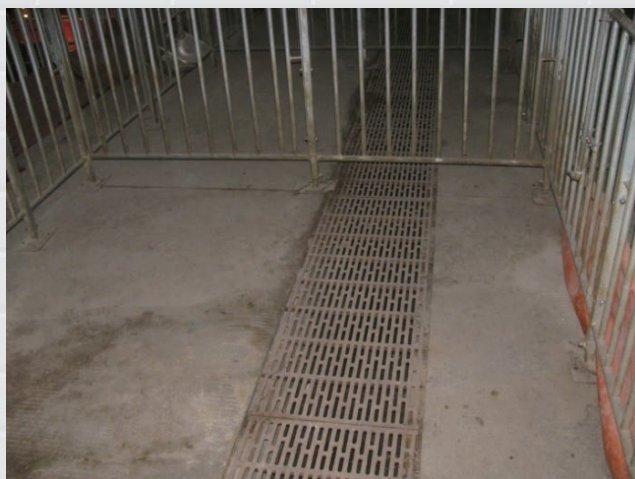
Covered nullah within pig barns for pig waste collection and drainage
