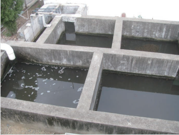
Wastewater filter and disposal system
