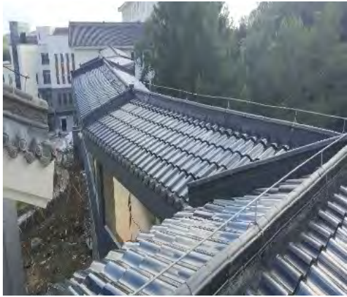
Photovoltaic tile project of a nursing home in Jilin 吉林養老院光伏瓦項目
