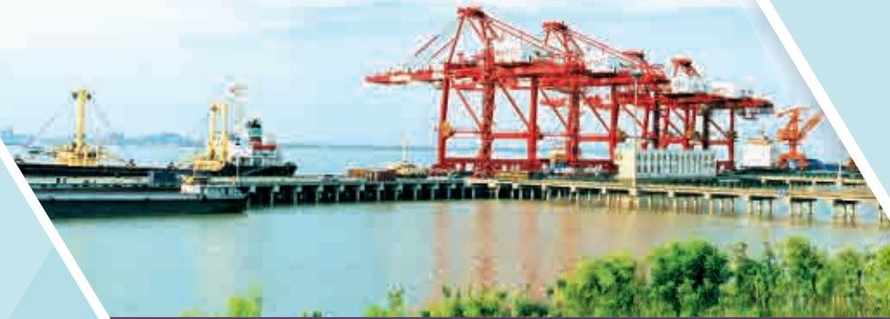
JIANGYIN SUNAN CONTAINER TERMINAL 江陰蘇南集裝箱碼頭
