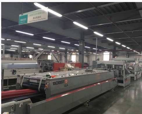
Complete replacement of LED lights 全面更換LED燈
