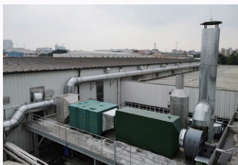
VOCs and ammonia collection and treatment system VOCs及氨氣收集處理系統
