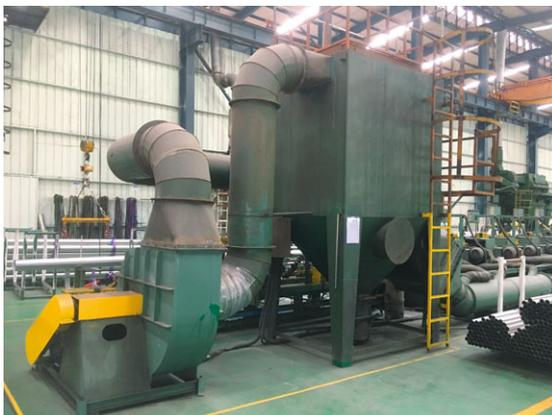
In order to effectively prevent and control dust pollution, improve air quality and protect public health, Guangzhou Mayer's production plants are equipped with dust collectors with pulse jet filter bags, which adopt automatic dust cleaning devices to maintain the stable filtering effect of the dust collectors and thus to reduce particles and dust emissions during production.
