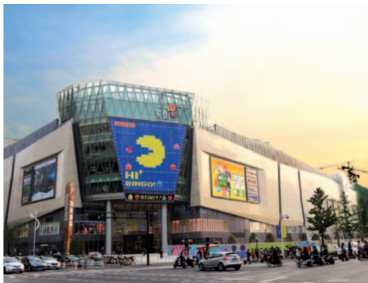
杭州濱江天街1期 Hangzhou Binjiang Paradise Walk Phase I
