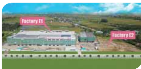
Vietnam Factory E (Under Construction) 越南E廠 (興建中)
