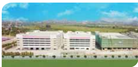
Vietnam Factory D (Under Construction) 越南D廠 (興建中)
