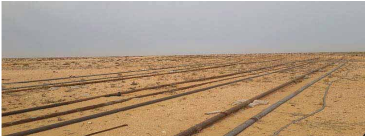
Figure AIII.3: Pipeline Installation
