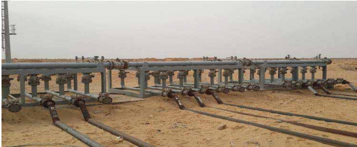
Figure AIII.2: Manifold
