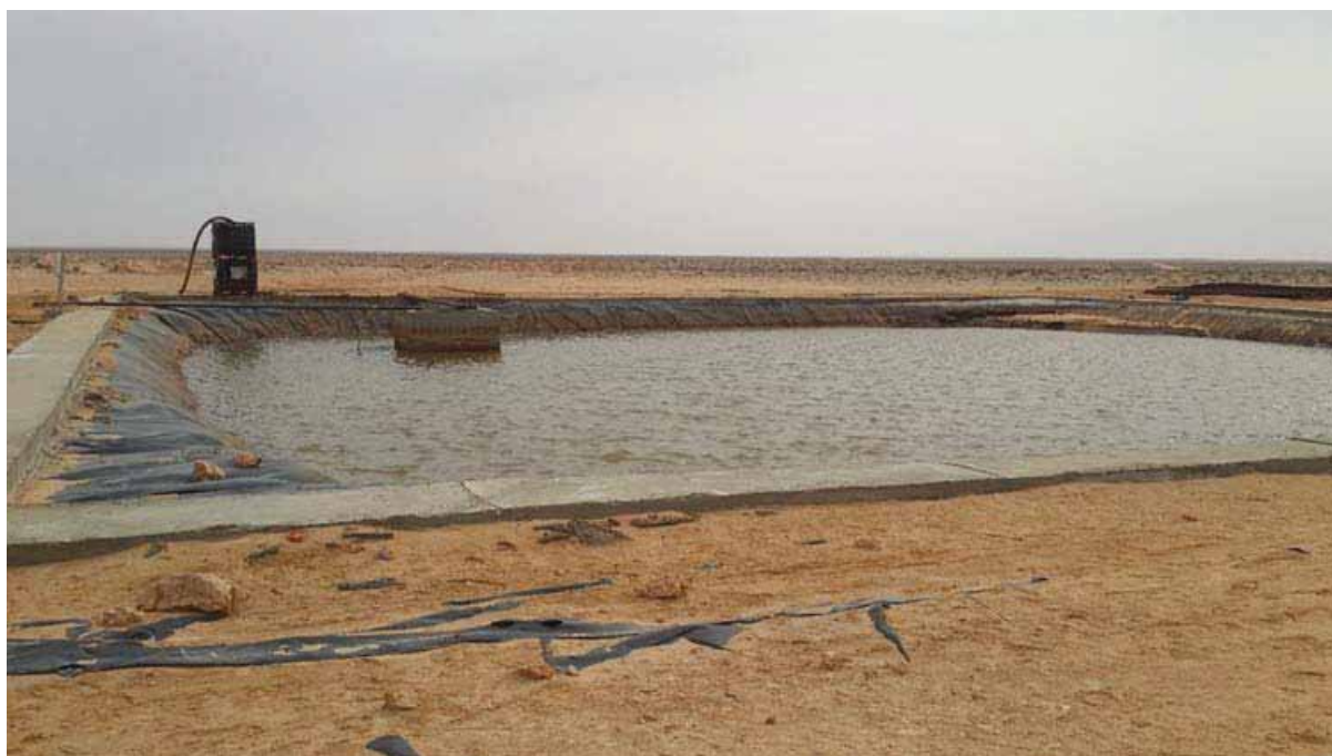
Figure AIII.8: Produced Water Lagoon
