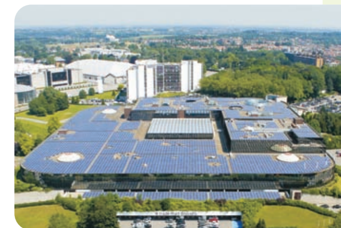
Largest rooftop solar farm in Belgium
