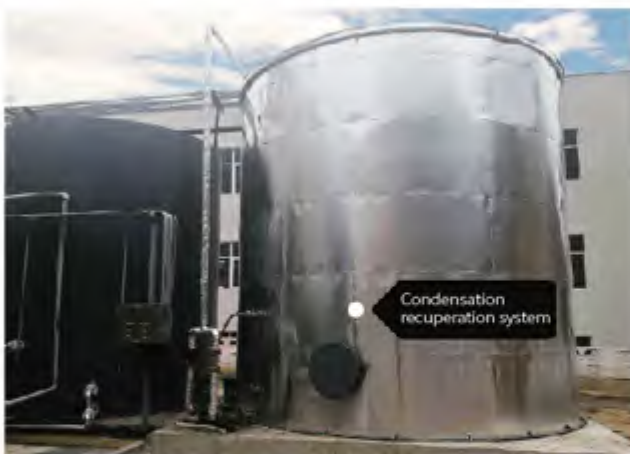
In 2018, China operations have invested in and transformed their wastewater system in the molybdenum-tungsten recovery facility. We built a condensation recuperation system in order to send the condensed water for storage pending reuse in production. Capable of recovering 80% of the condensed water, the system allows us to reduce the use of fresh water by 40 000 m 3 per year.
