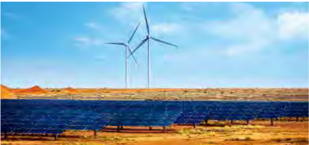
Energy Developments' Coober Pedy Renewable Hybrid Project powers the remote town of Coober Pedy with a hybrid of wind generation, solar generation, battery and other integration technologies.
