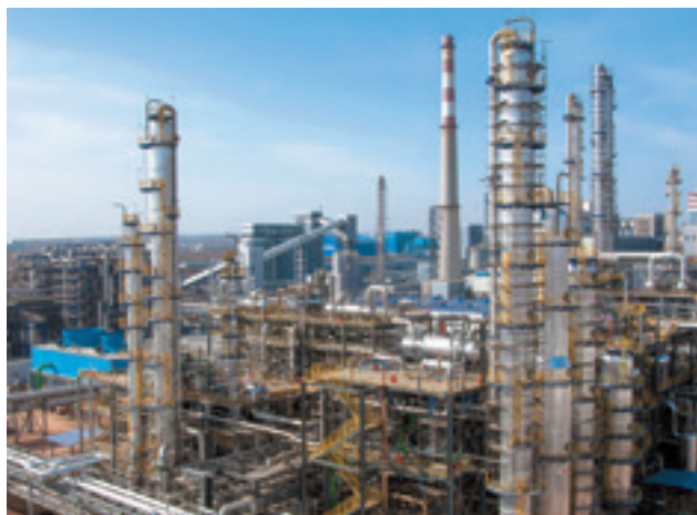
Clean coal chemical plant in Ordos, Inner Mongolia
