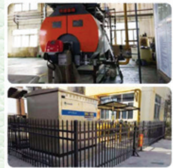
Natural gas boiler and gas pressure regulator
