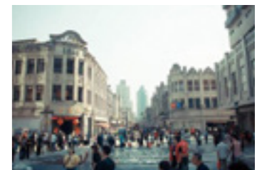
改造後蟬街風採 Chan Street after the renovation
