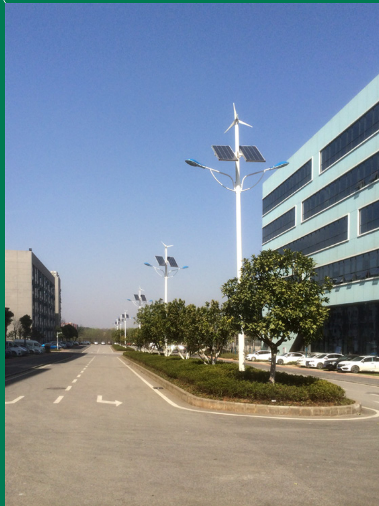
Solar panels and wind turbines provide renewable energy for all street lamps at the Wuhan Jewellery Park 太陽能板和風力渦輪為武漢珠寶文化產業園的所有街燈提供可再生能源
