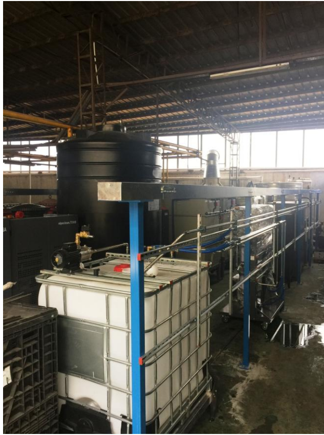
Sewage treatment system
