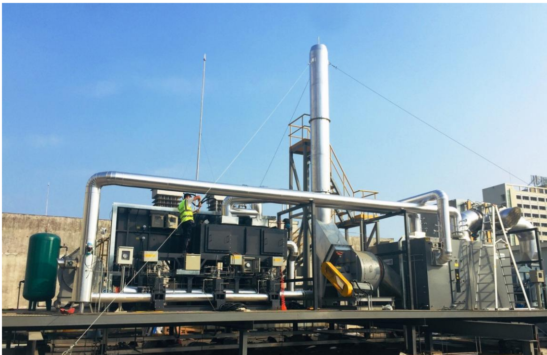
Upgrade VOCs equipment
