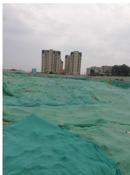
Covering exposed loess on site
