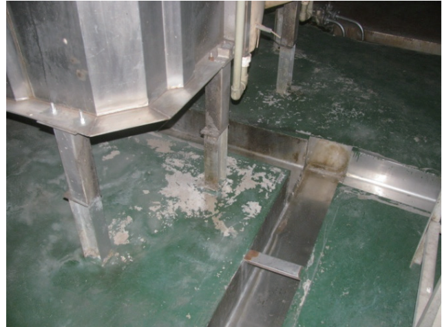
Gutters within slaughterhouse for waste water drainage
