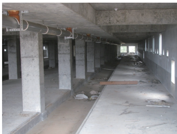
Construction of nullah within pig barns
