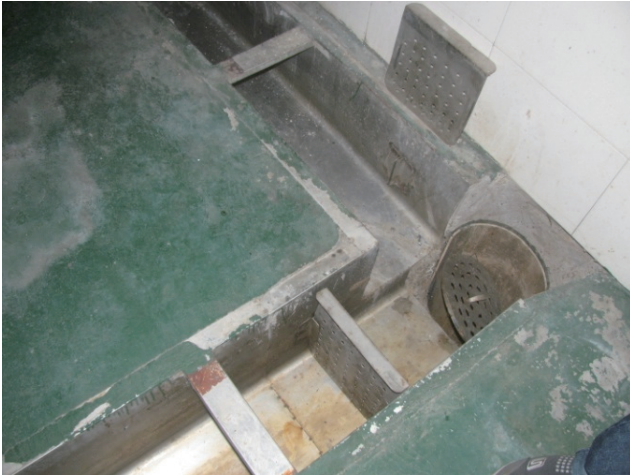
Gutters within slaughterhouse for waste water drainage
