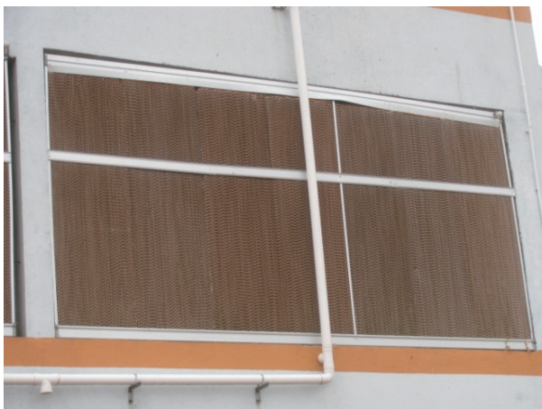
Evaporative cooling pad installed in the external wall openings
