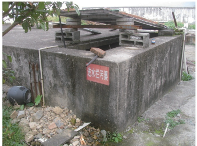
Wastewater filter and disposal system
