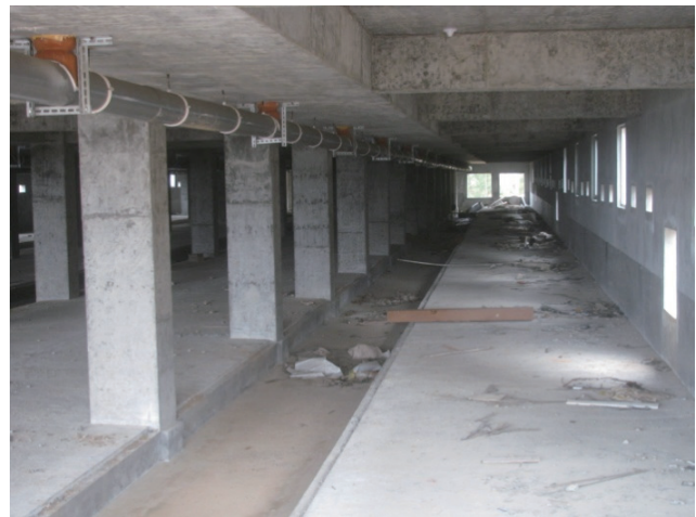
Construction of nullah within pig barns
