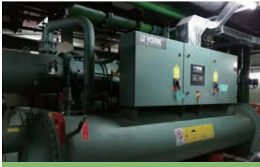
Ice-storage Air-conditioning Retrofitting
