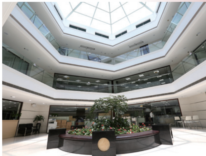
Glass ceiling design is adopted to maximise natural lighting in the office building of the factory area. 工廠區的辦公樓使用玻璃頂部設計，盡量利用天然採光。
