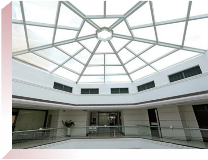
Glass ceiling design is adopted to maximise natural lighting in the office building of the factory area. 工廠區的辦公樓使用玻璃頂部設計，盡量利用天然採光。
