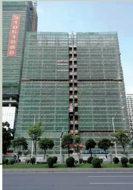
Substantially completed commercial building at Guangzhou South High Speed Train Station 位於廣州高鐵南站的商業大樓已封頂
