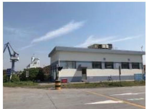
Electric power supply room – After removal of rust and new paint work
