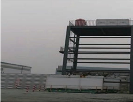
New fire system – water tanks and pump
