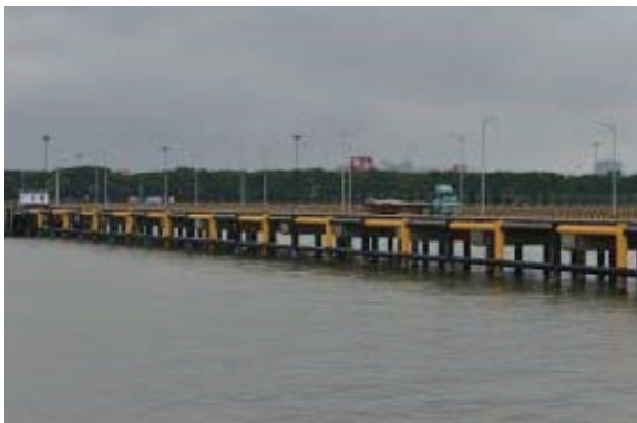
Railing – After removal of rust and new paint work
