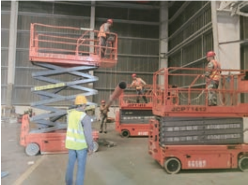
New fire system – installation of fire hose
