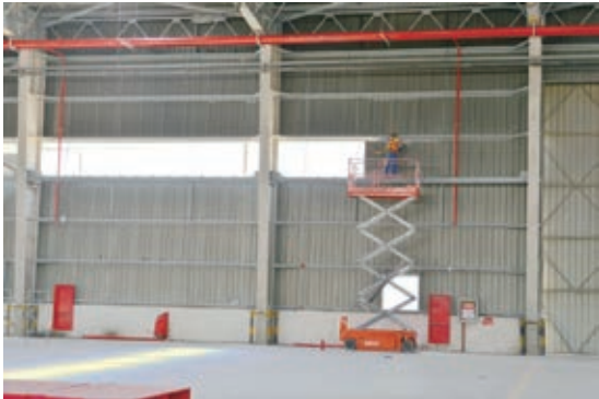
New fire system – fireproof coating
