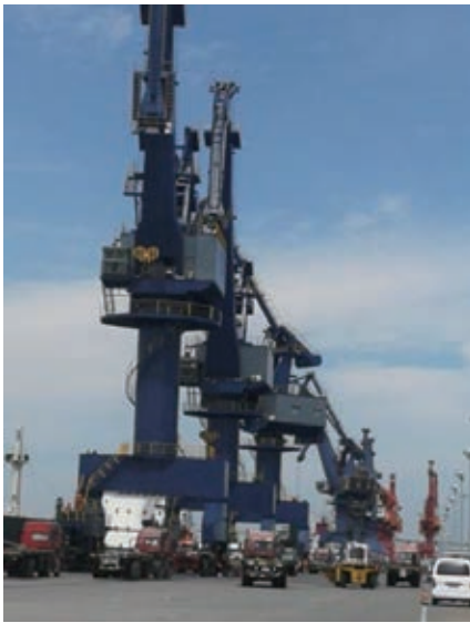
Shore cranes after removal of rust and new paint work
