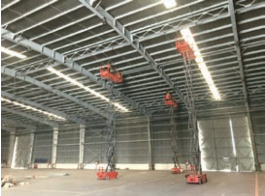
New fire system – installing air sampling system, fire retardant hose
