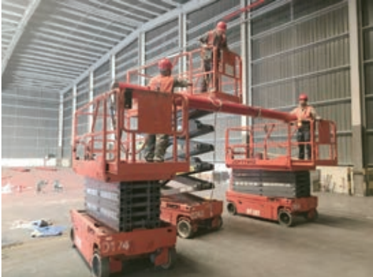
New fire system – installation of fire hose
