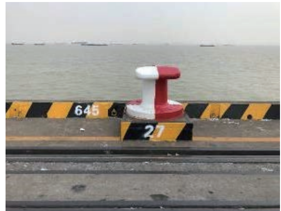
Bollard – After removal of rust and new paint work
