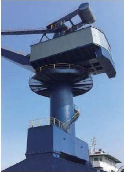
Shore cranes after removal of rust and new paint work
