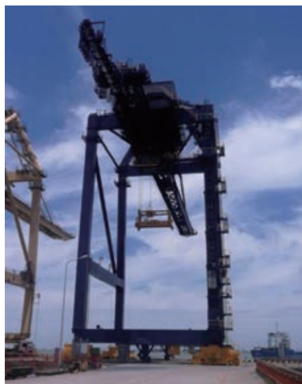
Quay cranes after removal of rust and new paint work
