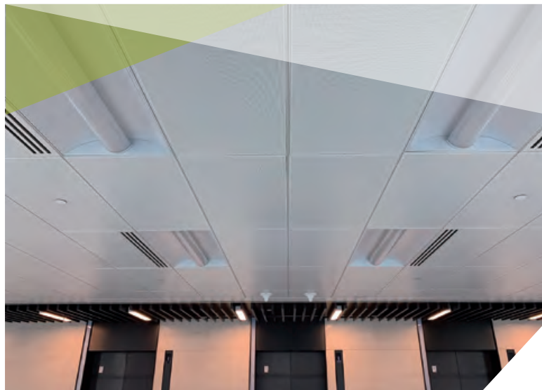
Supply and installation of suspended ceiling system for proposed office development at 1 Hennessy Road 軒尼詩道1號之建議辦公室發展項目－供應及安裝假天花系統
