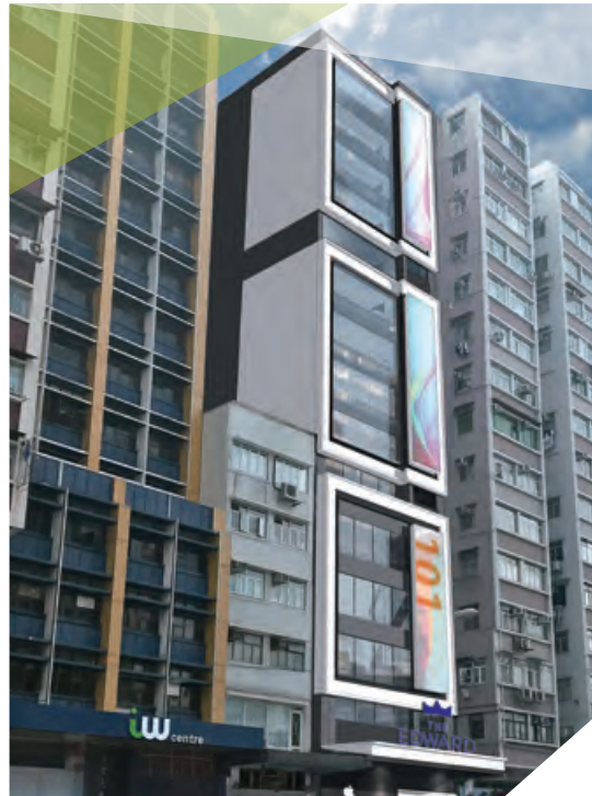
The Edward at 99-101 Lai Chi Kok Road (rendering of the development) 位於荔枝角道99號至101號之The Edward (設計概念圖)
