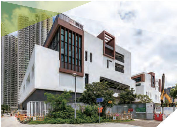
30-classroom secondary school at Site 1A-2, Kai Tak Development 啟德發展區1A-2地盤之一所30班房中學
