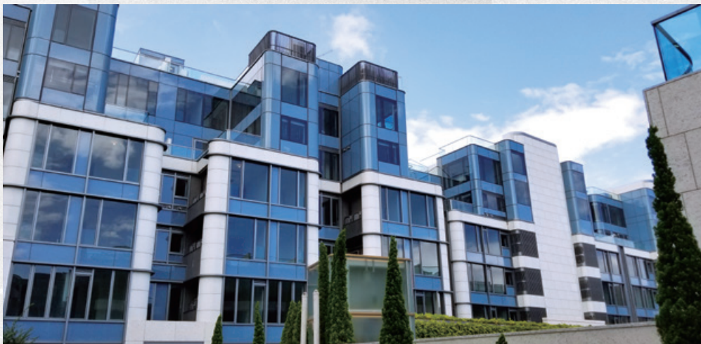
Residential development at STTL 567, Lai Ping Road in Area 56A, Kau To Shan, Shatin, New Territories 新界沙田九肚山56A區麗坪路沙田市地段第567號之住宅發展項目
