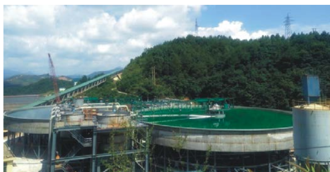
Environmentally friendly treatment system for copper-containing acidic water of the Zijinshan gold and copper mine at a capacity of 30,000 cubic metres/day
