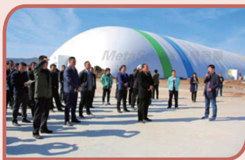
External view of air dome plant 氣膜廠房外觀圖
