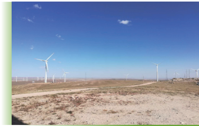
Wind Power Plant, Baotou city, the Inner Mongolia Autonomous Region 內蒙古自治區包頭市風力發電站
