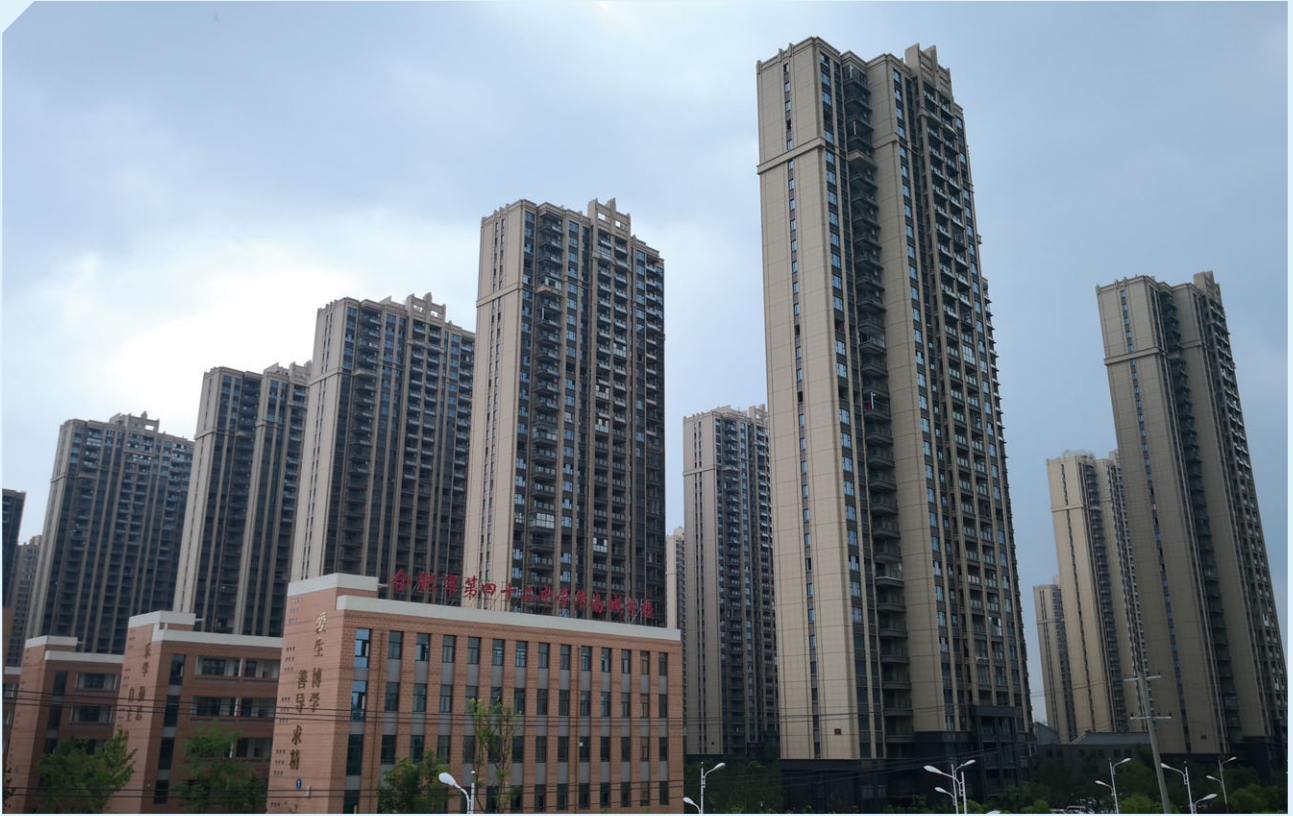
Residential ancillary (Zijingmingdu) and the secondary school in CSC Hefei 於合肥華南城的住宅配套紫荊名都及中學
