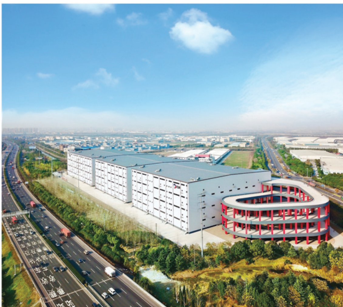
Jiangsu Friend—III (China) (directly owned by us) is a multi-story ramped distribution center located in Jiangsu Province. Completed in 2017, this facility is four stories tall and has a GFA of 206,418 sq.m.
