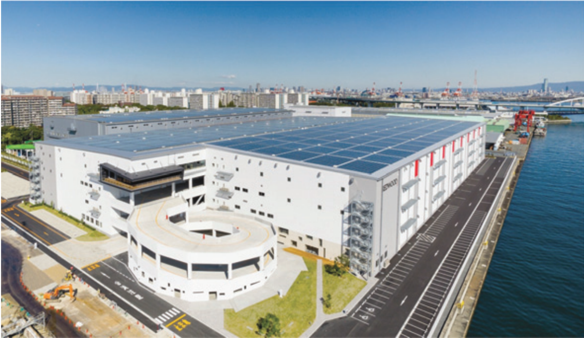
Nanko—I (Japan) (owned by a fund managed by us) is a double-ramped multi-story distribution center strategically located at the port of Osaka. Completed in 2016, this facility is four stories tall and has a GFA of 125,813 sq.m.
