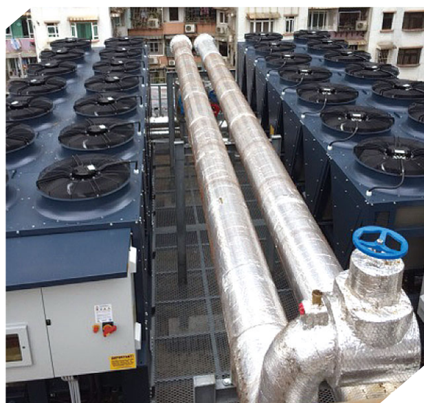
Magnetic bearing oil-free chiller
