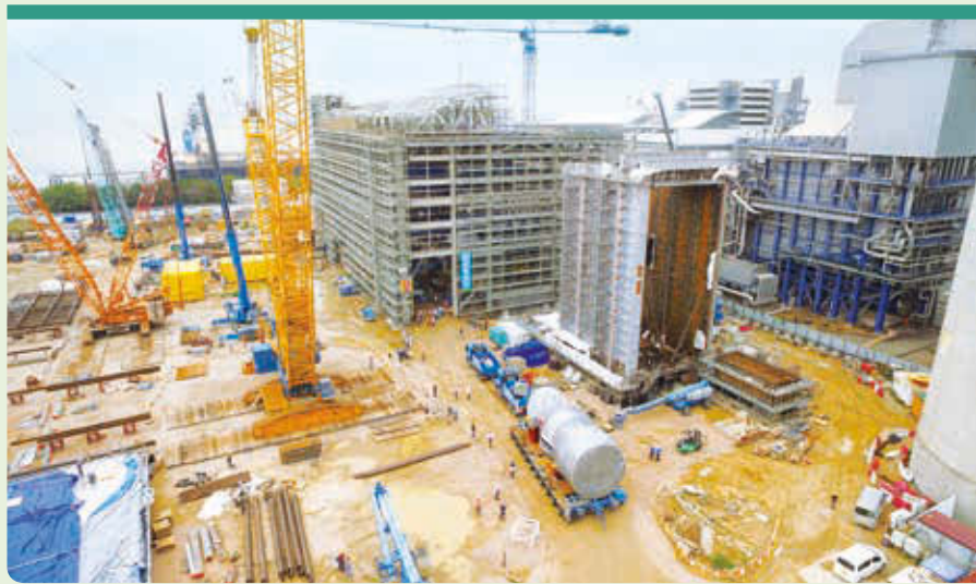
▲ Off-site fabrication allows construction to stay on track despite space constraints at Lamma Power Station.
