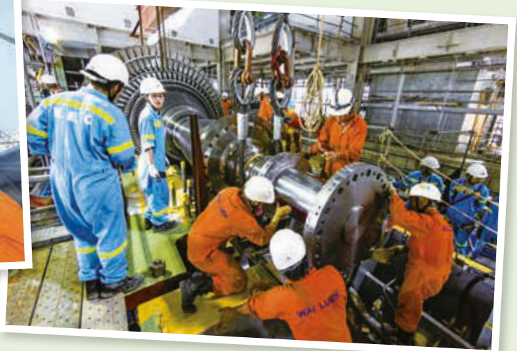
▲ Engineers are assembling steam turbine for L10 generating unit.
