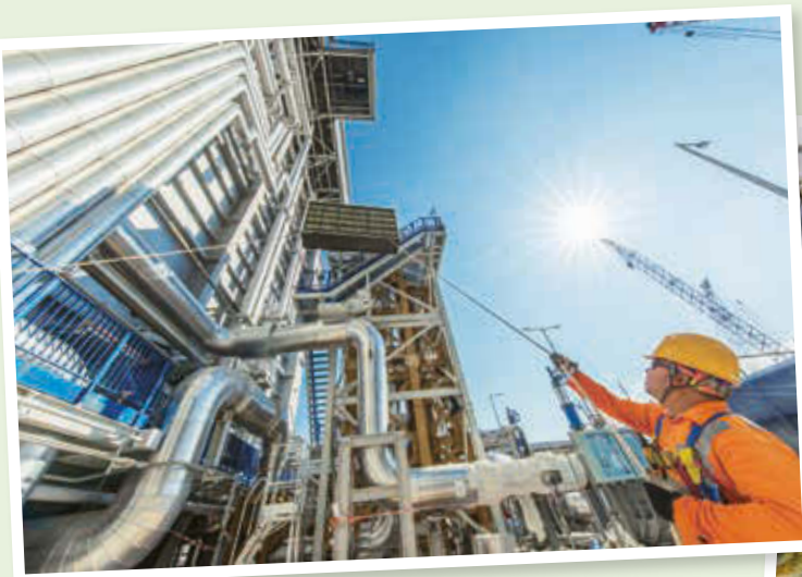
▲ Selective Catalytic Reduction System under installation.
