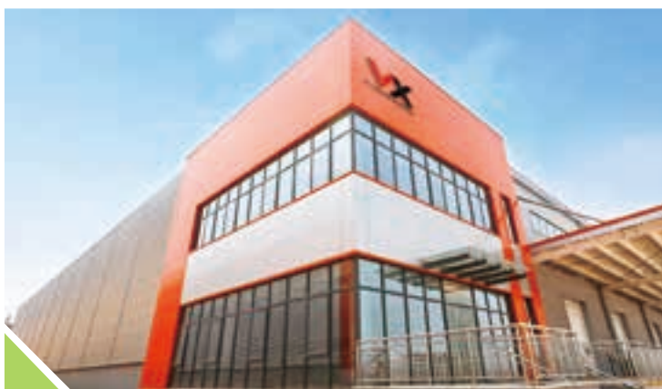
Wuhan Yangluo Warehouse
