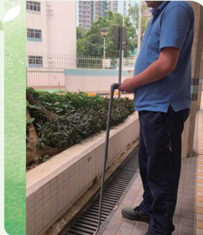
Demonstrating the application of the High-Pressure Sewer Cleaning Hose 展示高壓沖渠喉管的使用方法
