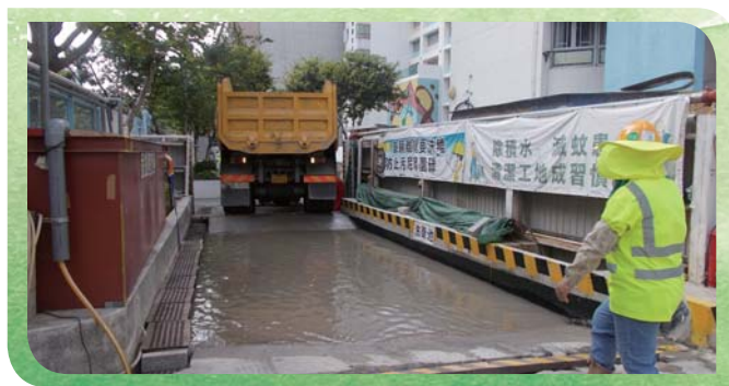
Wheel washing for air pollution control 清洗車輪以控制空氣污染
