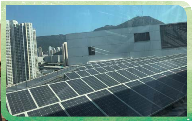
The rooftop viewing gallery of EMSD headquarters with over 2,000 photovoltaic panels 機電署總部的屋頂觀景台設有2,000多個太陽能板
