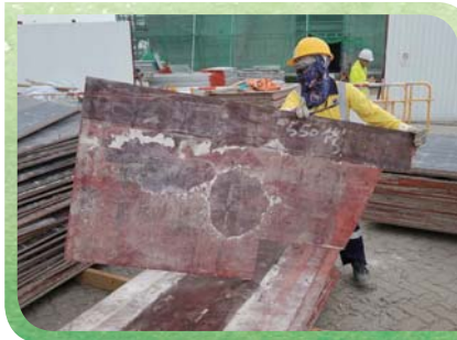
Our specialist handled and removed nailed wood with precautions 我們的專系工人謹慎地整理和拔木釘
