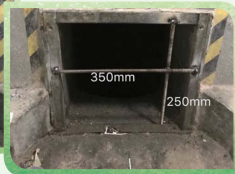
Reduction the size of refuse chute gate 減少了垃圾槽槽口門
