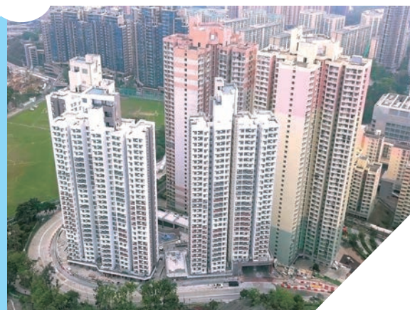
Construction of Home Ownership Scheme Development at Sheung Lok Street, Homantin 位於何文田常樂街 興建居屋發展項目 ▶
