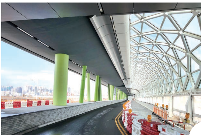
◀ Kai Tak Development - Stage 2 Infrastructure Works for Developments at the Southern Part of the Former Runway 啟德發展計劃 — 前跑道南面第2期的基礎設施發展工程
