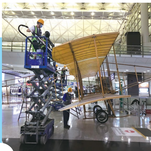
▶ Hong Kong International Airport Term Contract M297-4 Maintenance, Improvement and Refurbishment Works for Buildings 香港國際機場定期合約M297-4樓宇保養、改善及維修工程
