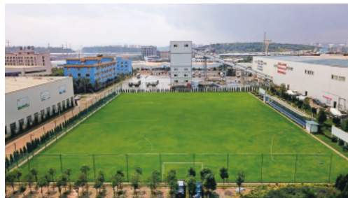
Plant green area 廠區綠地
