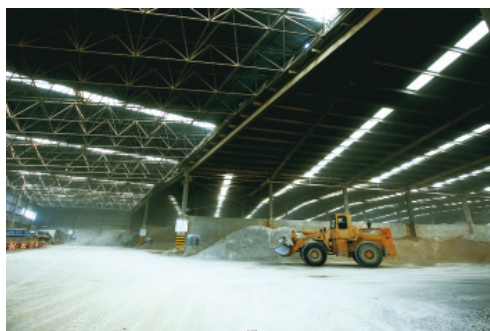
Stockyard with spraying system 裝有噴淋系統的料場環境
