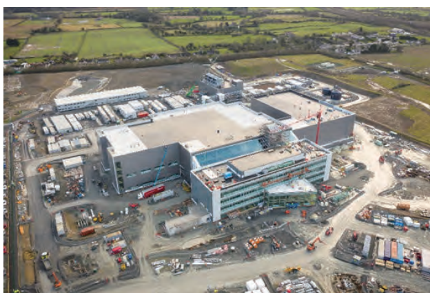
Latest construction progress of our Ireland Site
