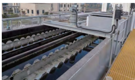
Sewage treatment plant of Wuxi Site
