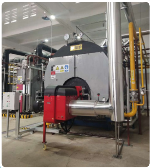
合肥統一鍋爐低氮改造 Modification of the boilers in Hefei President with low-nitrogen technology
