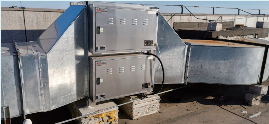
FNT-JD-16A 型靜電式飲食業油煙淨化設備 FNT-JD-16A electrostatic catering fume purification equipment
