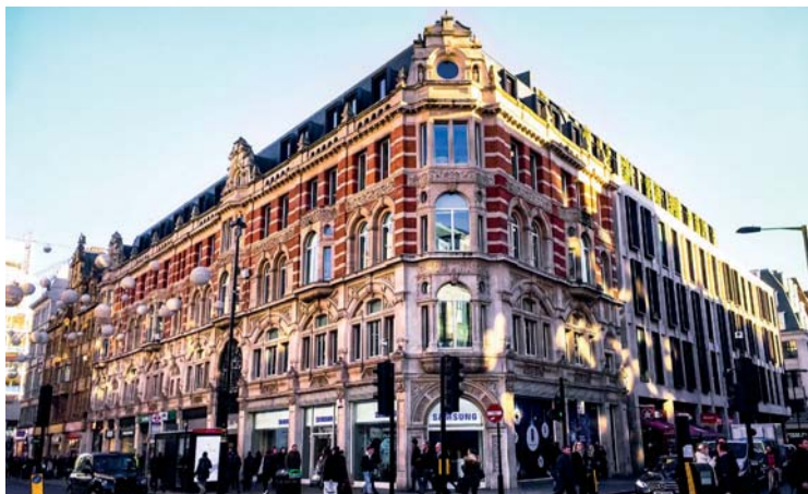
Ampersand Building, London 倫敦Ampersand大廈
